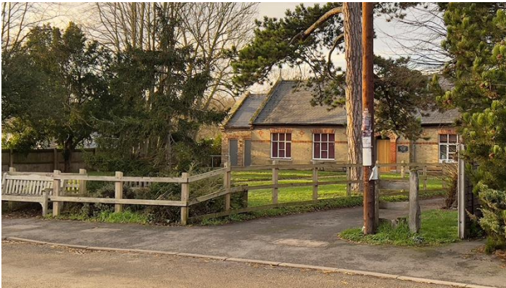
White House opposite with Car Park sign (From South)
